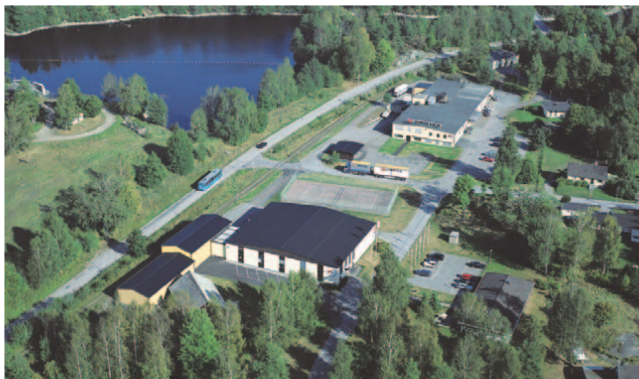
Partex Head Office and production plants in Gullspång Sweden.
